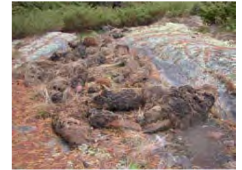
Bear Damage to paths
