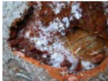
Bark damage and decay
