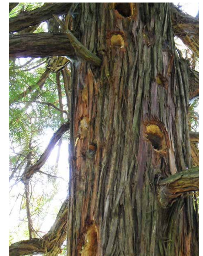
Below: Note extensive pileated woodpecker damage to venerable nearby cedar tree, revealing hollow core
