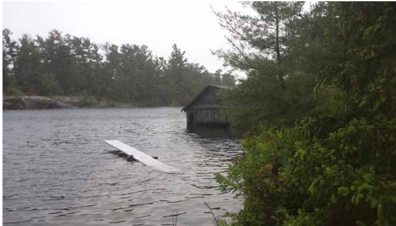
Throughout the summer season of 2020, extreme fluctuations of water level extending from 16" (400mm) above the high water benchmark to 12" (300mm) below have been witnessed. Archers Bay was particularly active with water seching in and out in constant cycles. The water extended far inland almost cutting off parts of OK Point and extending into the Troll Bridge Gulch. The Giants Causeway on the north side was often underwater.
